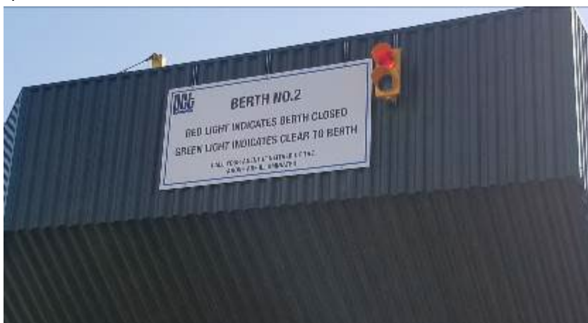
Photo 4: Berthing indicator light located on the chute storage tower at the east end of berth 2.
