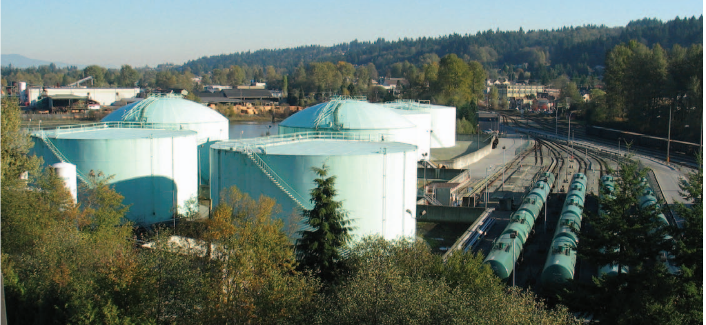
Ethylene glycol is stored for shipment in sealed tanks, which altogether can hold up to 53,000 metric tonnes.
