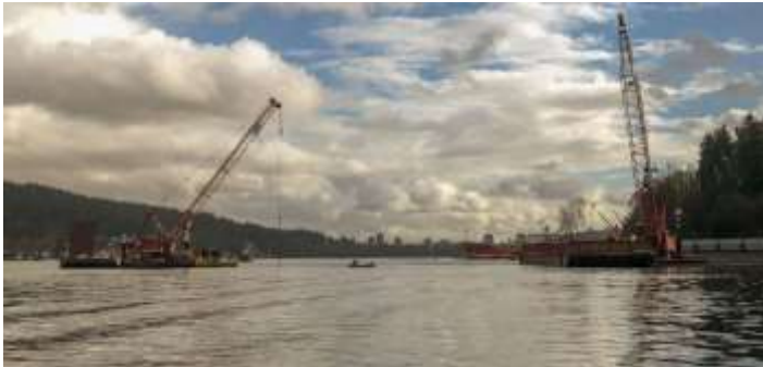
Pipeline removal derrick (left) and PAH dredge derrick (right) working safely in proximity near Reed Point
