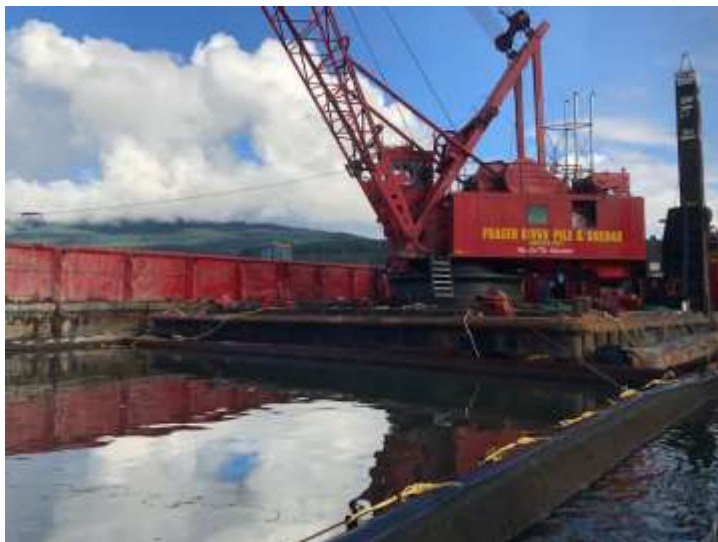
Mackenzie derrick using silt curtain for turbidity control and placing PAH affected sediment into sealed scow.
